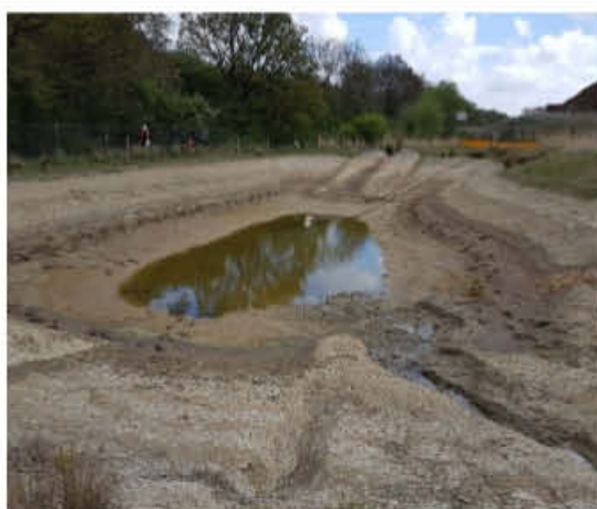
Photograph 11. Waterbody in northwest corner of ENRMF being drawn-down.
